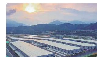
Qingxin Cloud Computing Center, in Qingyuan, Guangdong
