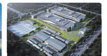
Data Centre Project in Johor, Malaysia
